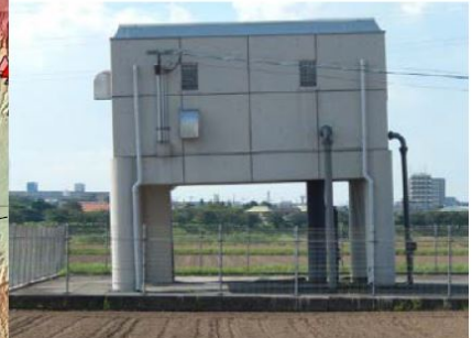
Tilted RC housing of pump for Akita clean water well No. 2 at N32.7670°, E130.7786 °: A low lying area east of this housing is found sunken by more than a meter
