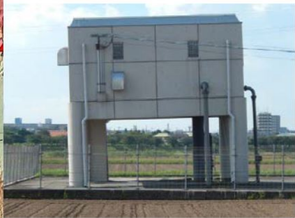
Tilted RC housing of pump for Akita clean water well No. 2 at N32.7670°, E130.7786 °: A low lying area east of this housing is found sunken by more than a meter
