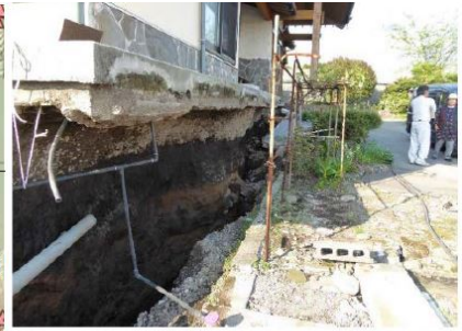
House hanging a little over the northwestern offset of the ground at N32.9568°, E131.0368
